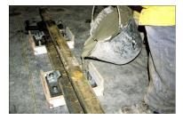
**RESOLTECH 2050E GRIS N ° 1 / 2059E** system is a filled epoxy casting system that allows any type of sealing or gravity levelling.
